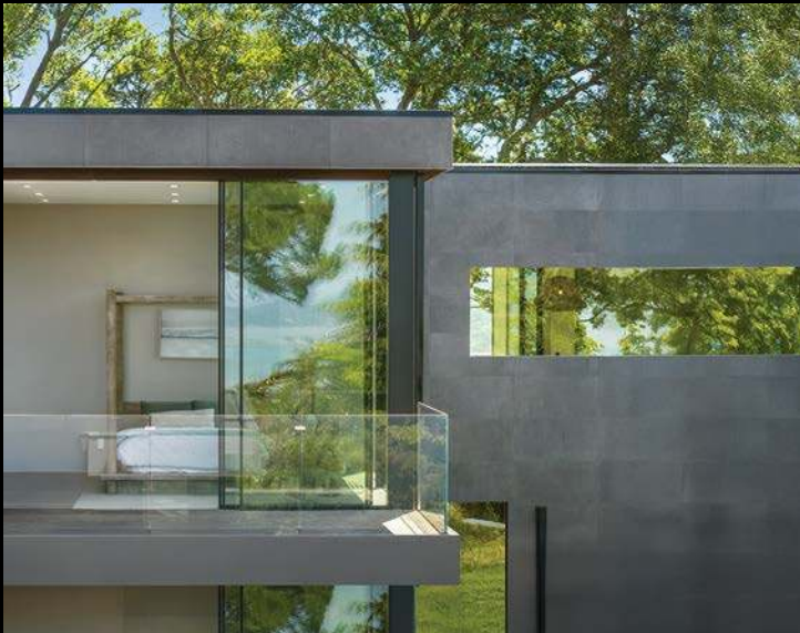
Jonathan Prewitt Photography | Murdock Architecture
