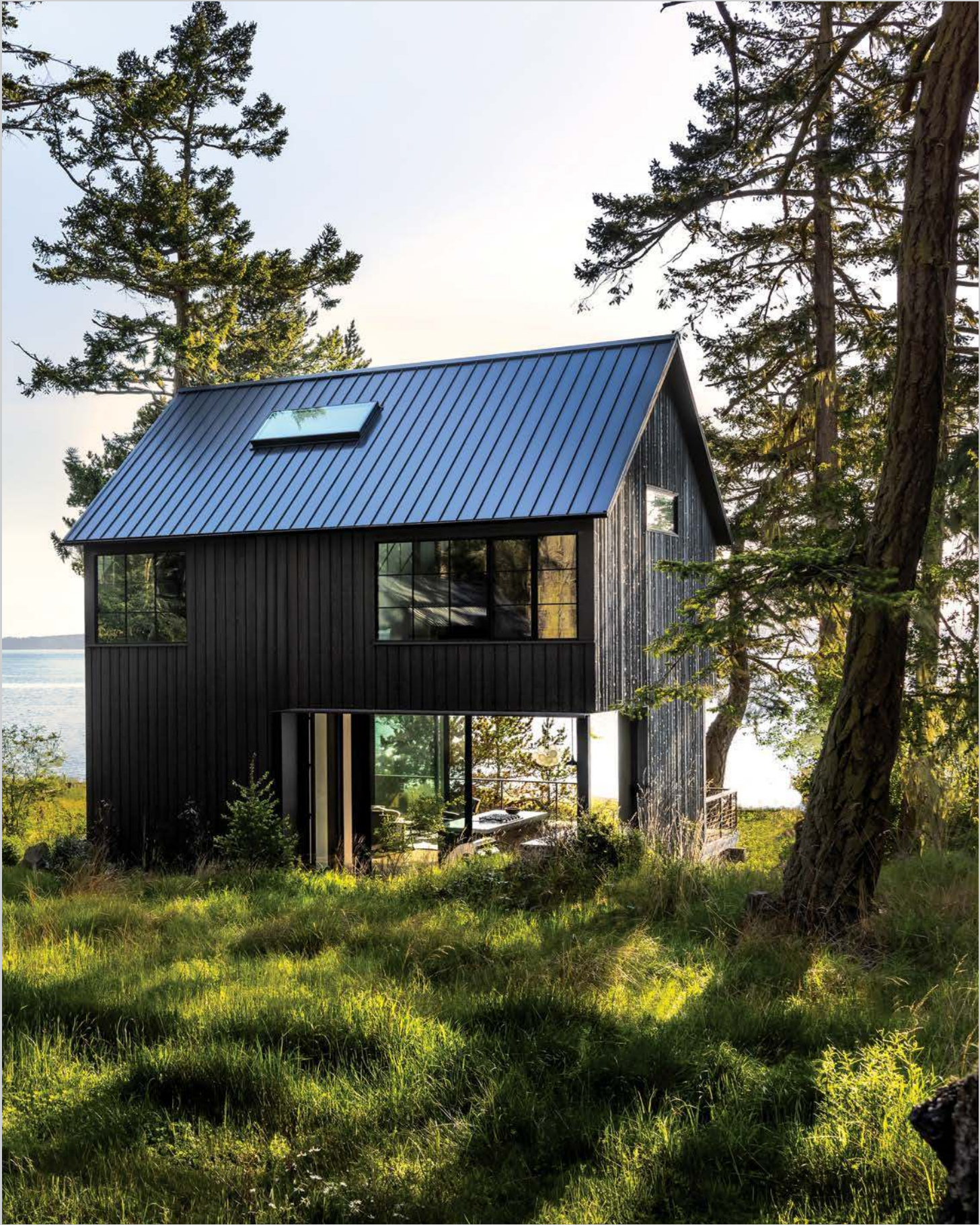
Taj Howe Photography | Heliotrope Architects | Tye Contracting
