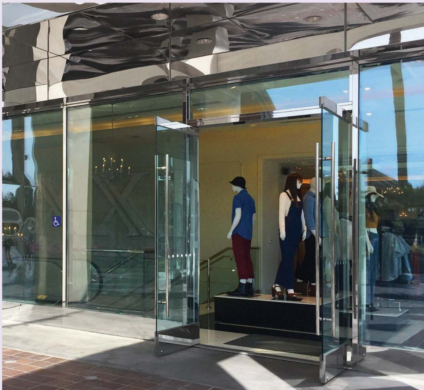
All Glass Entrance Doors with 1/2" x 7" Threshold
