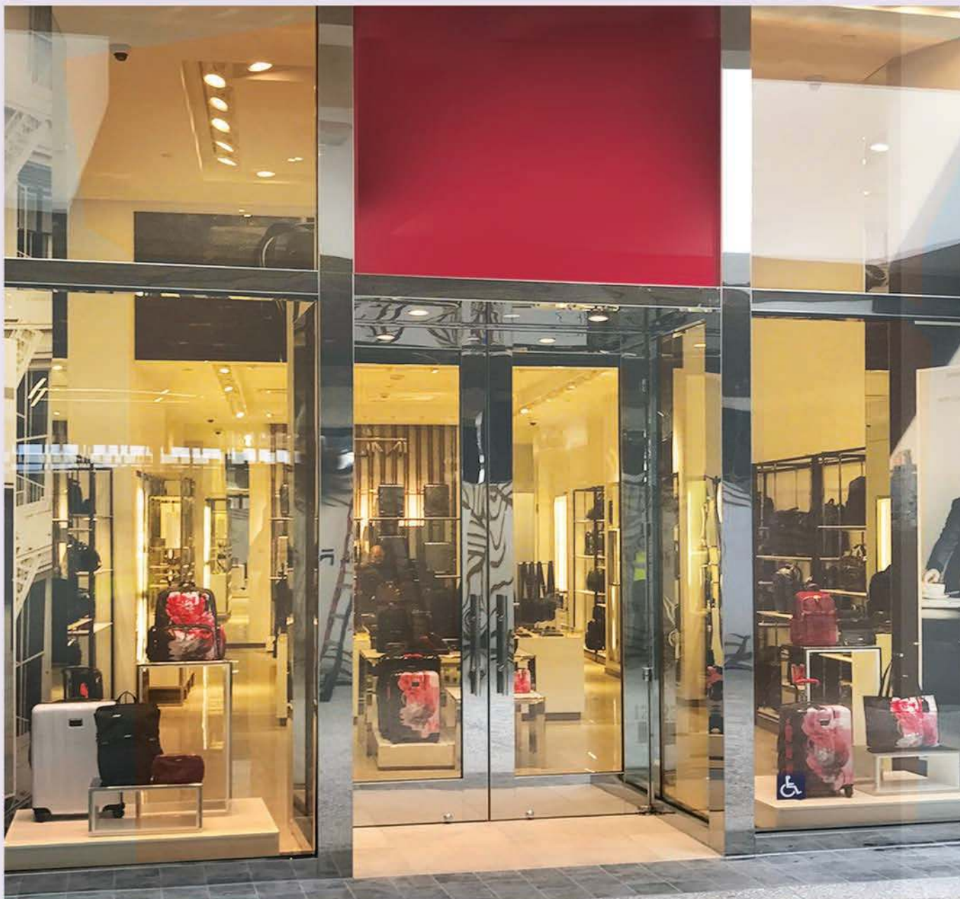
Full Frame Cladded Doors in Polished Stainless Steel
