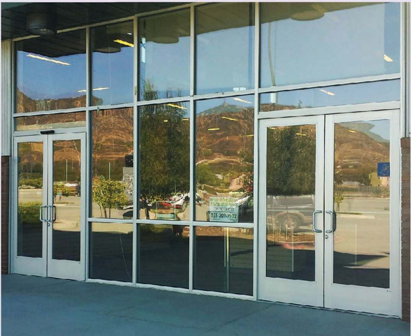
Complete Entrance System with PRL Fabricated Storefront , Doors & IG Units with Reflective Glass
