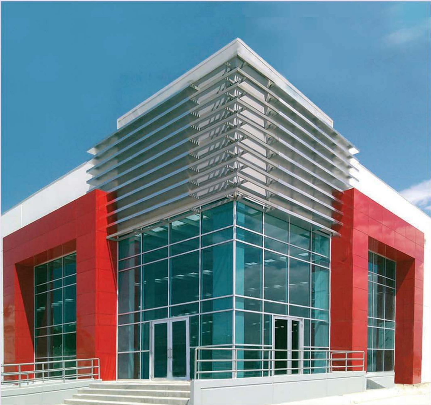
Curtainwall with 1/4" Solarban® 60 Low-E and Atlantica IG Units
