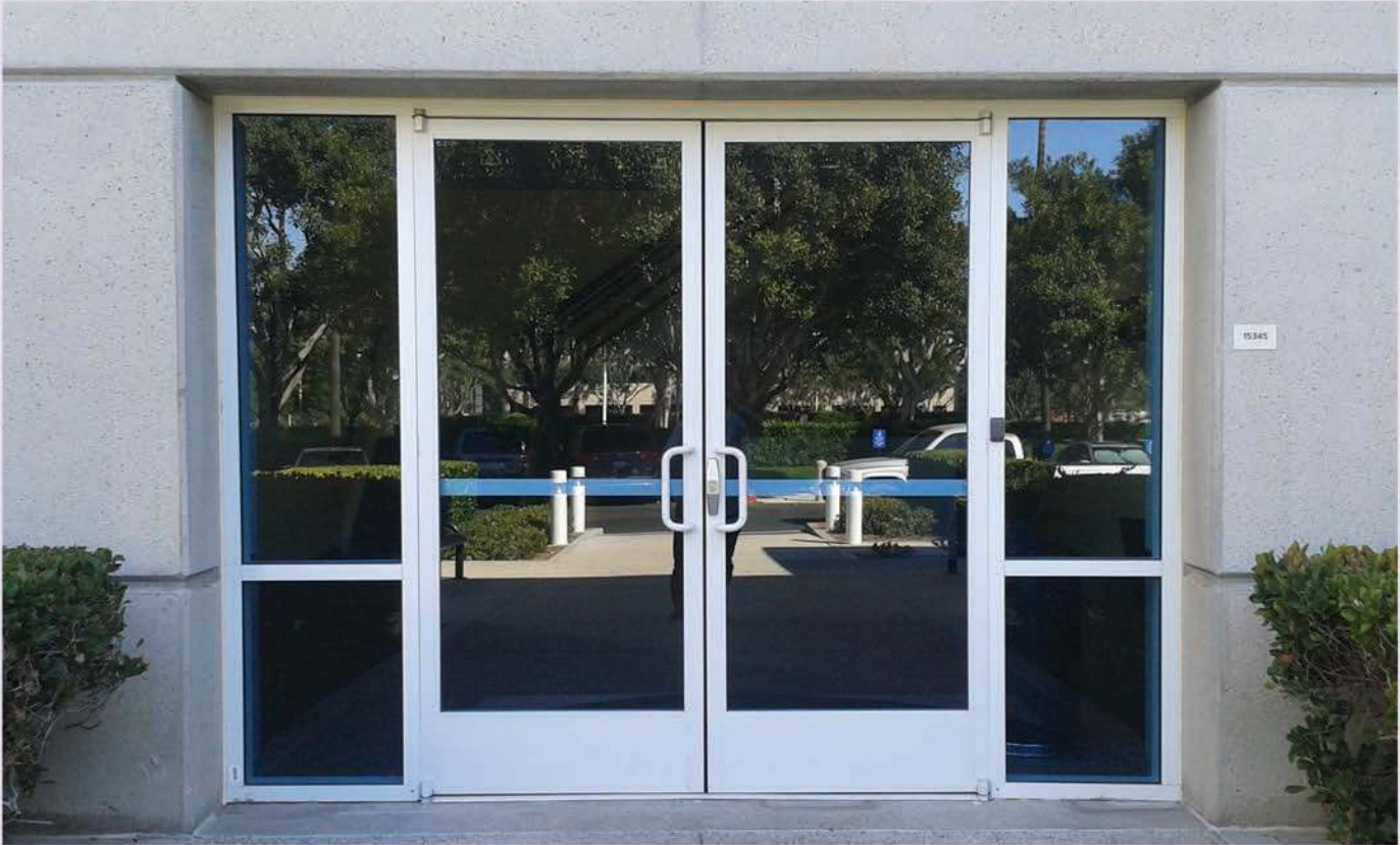
Double Aluminum Doors with Reflective Glass, Panic Hardware & PL-3 Offset Pulls
