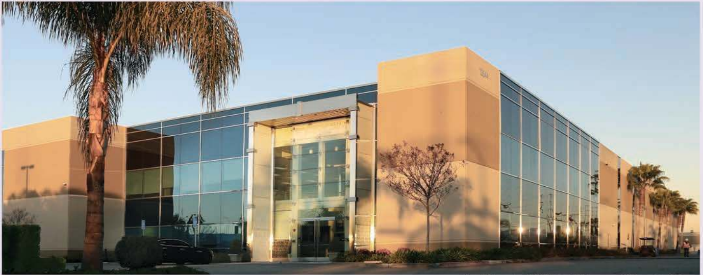
Curtainwall with Tinted Glass and Spandrel Glass
