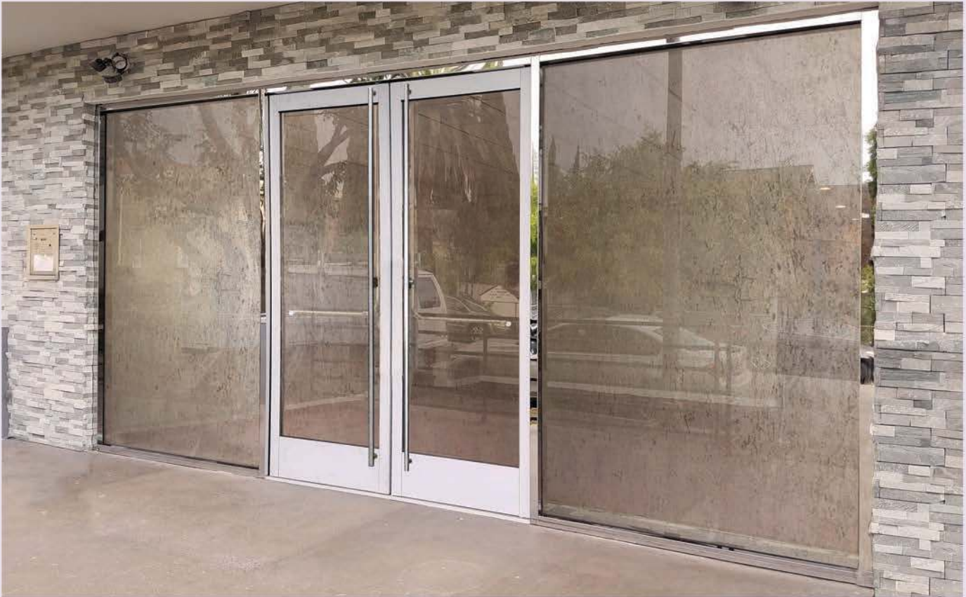
Medium Stile Full Frame Cladded Doors with PL-100FS Panic Device
