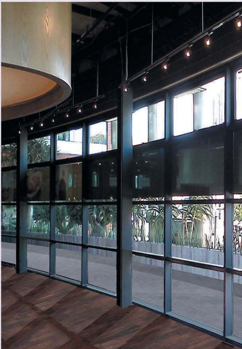
Curtainwall System with Reflective Glass
