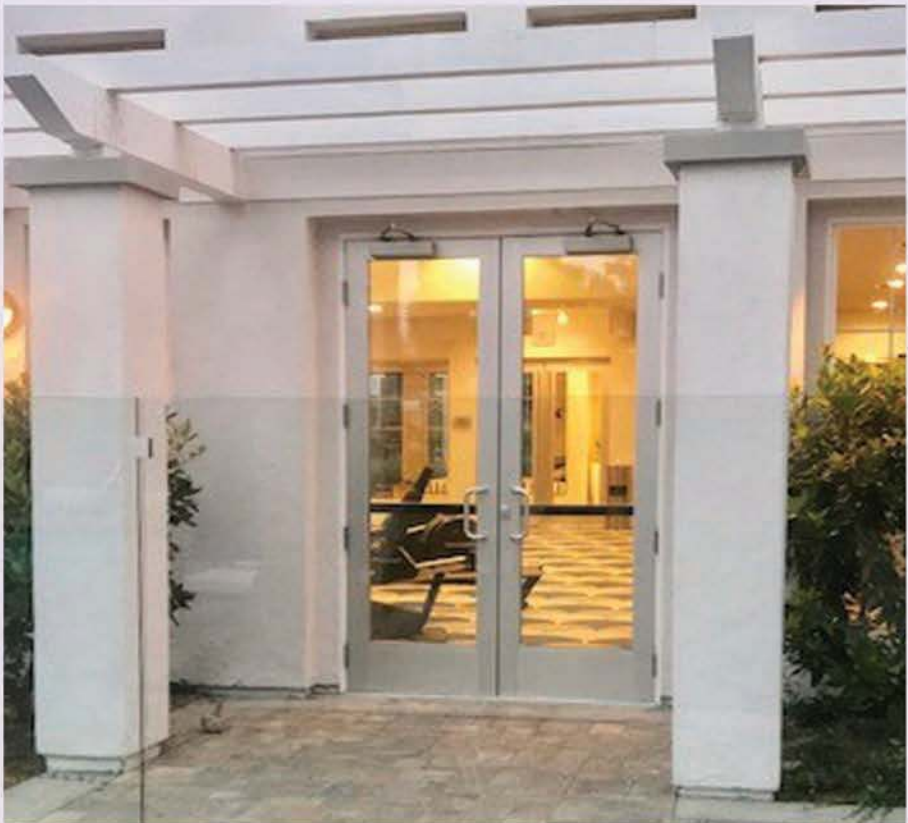
Aluminum Door with an Electric Strike and Offset Handle
