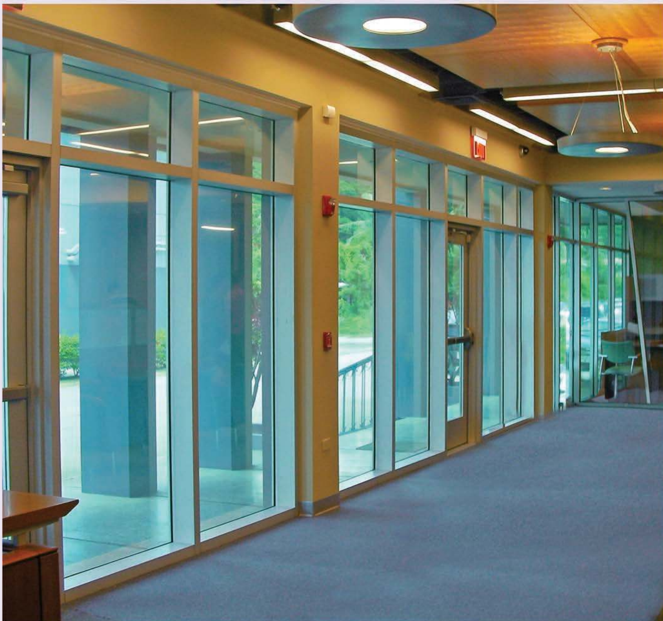
Aluminum Storefront system with IG Unit Clear Glass
