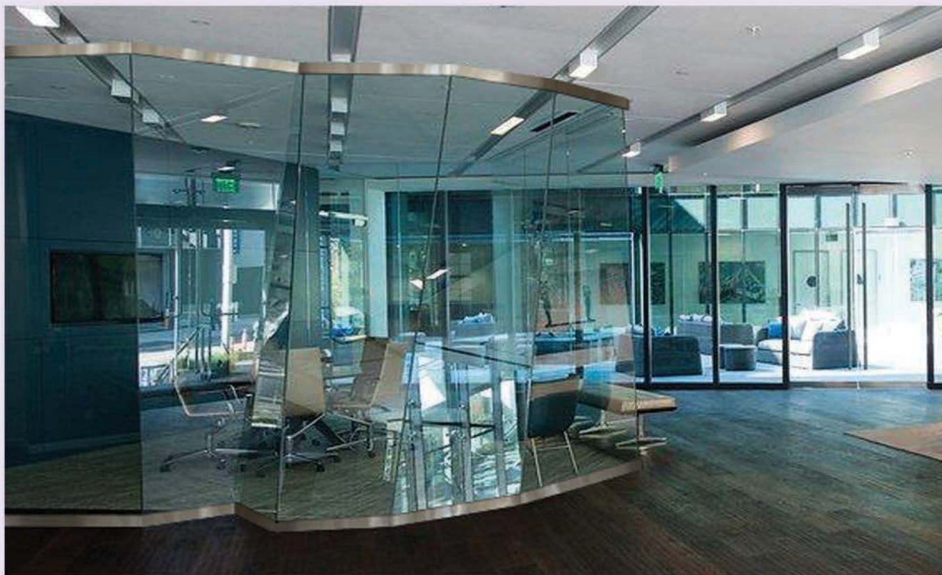
Conference Room with Custom Glass and Compound Angle Cladded Channels
