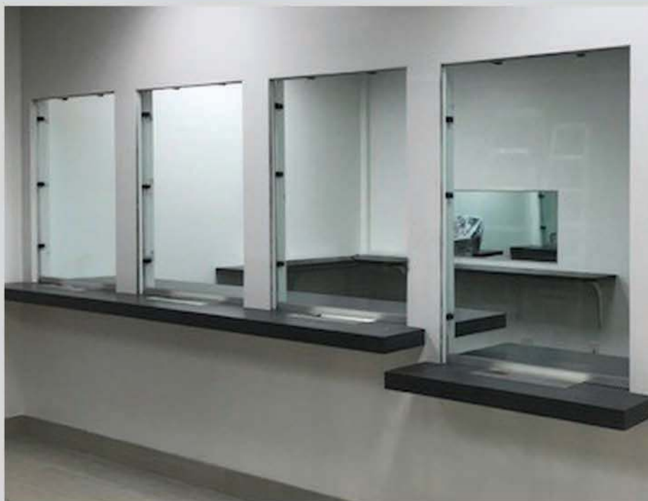
Transaction Windows with Level 1 Bullet Resistant
