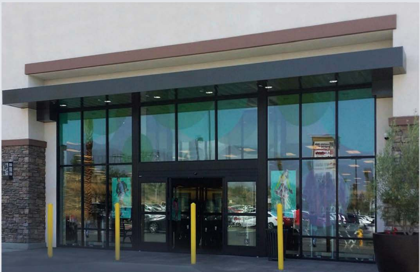
Aluminum Storefront with Reflective Glass IG Units
