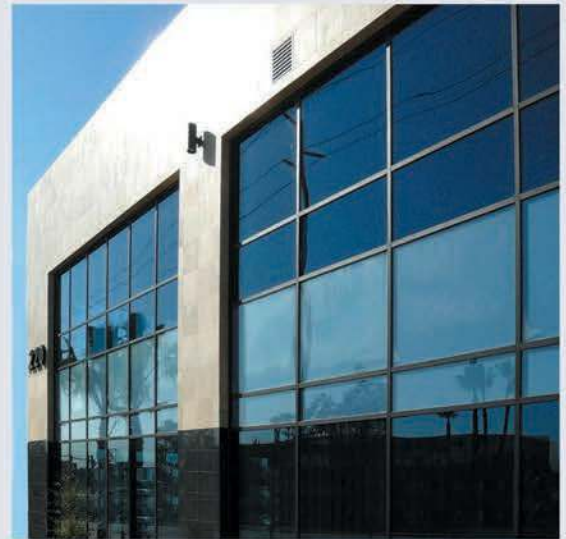
Curtainwall with Tinted & Spandrel Glass
