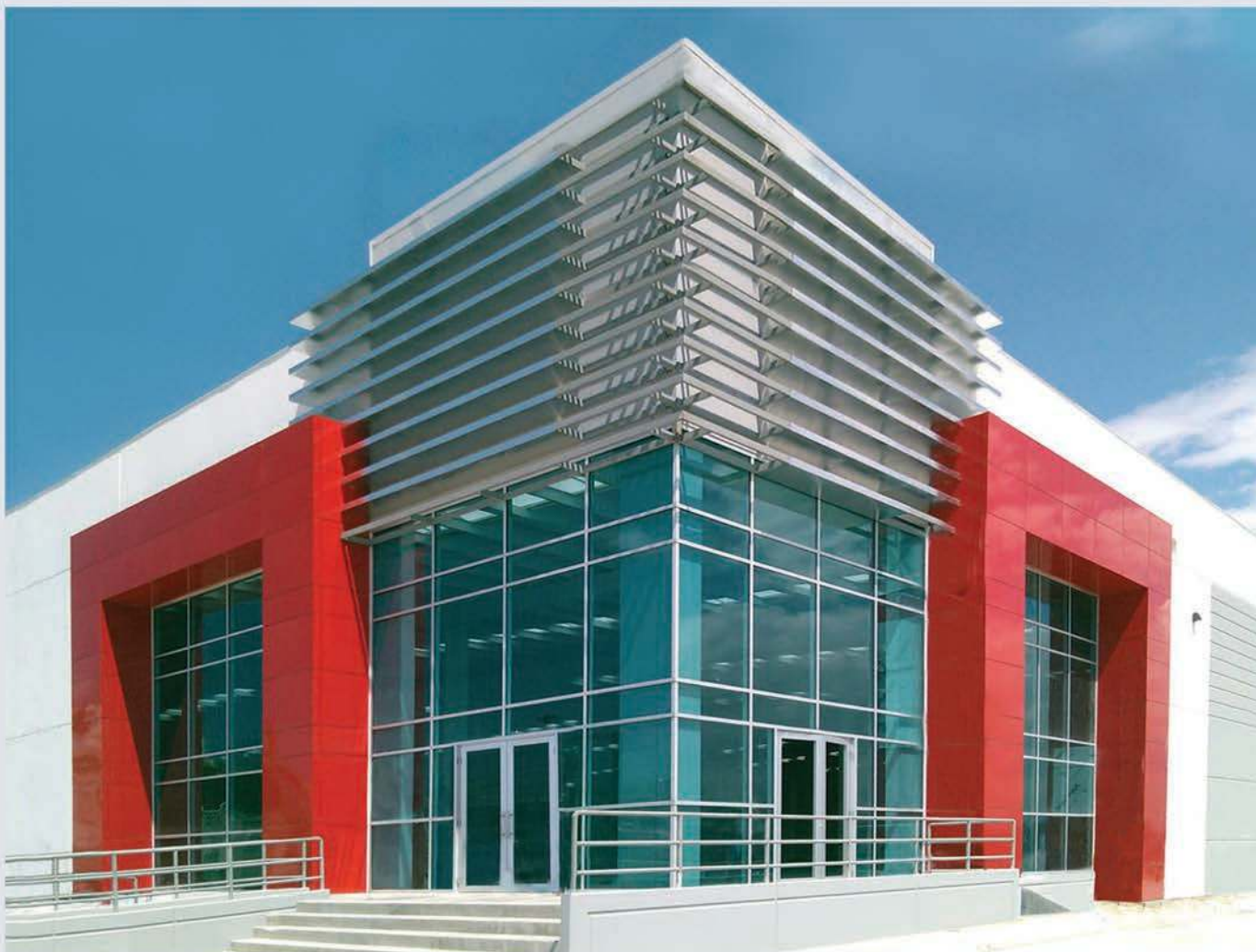
251 Series with Steel Stiffener Reinforced and 1/4" Solarban® 60 Low-E and Atlantica IG Units
