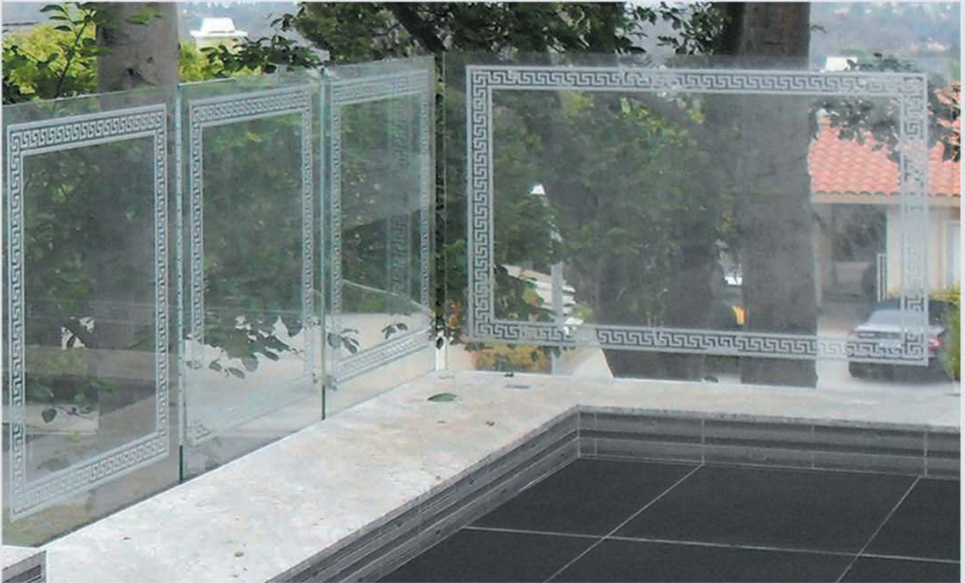
Handrail System with Custom Sandblast Border
