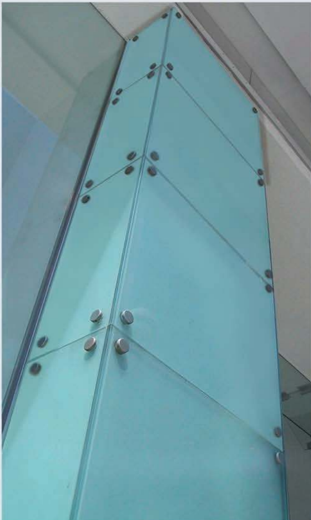
Spandrel Glass Panel Column Cover
